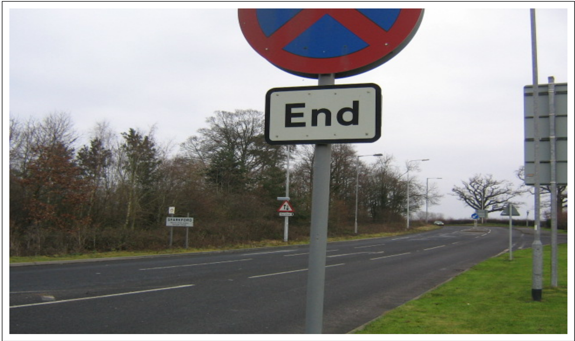
P0002 – Grey paint / coating to small sign post at filling station access road
