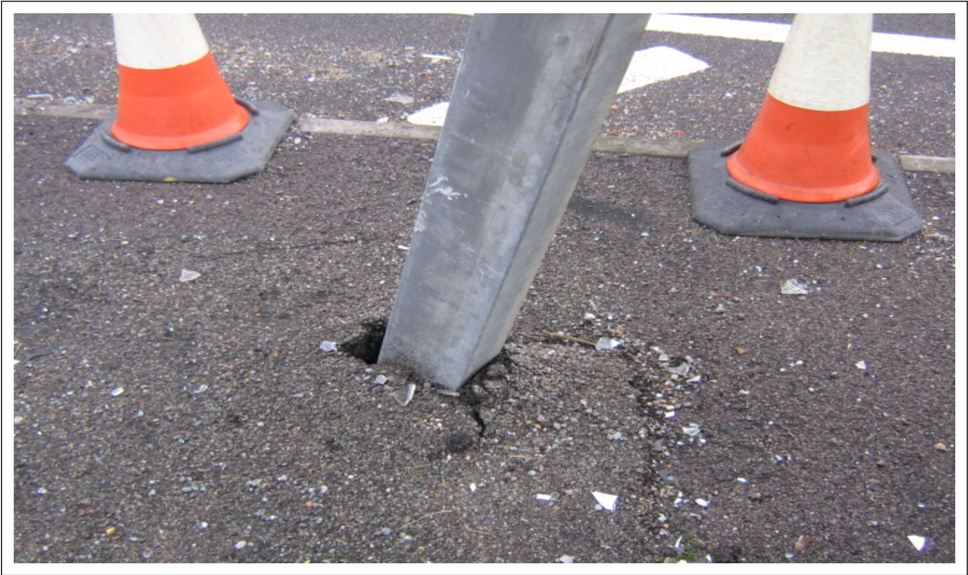
P0004 – Surfacing to island area
