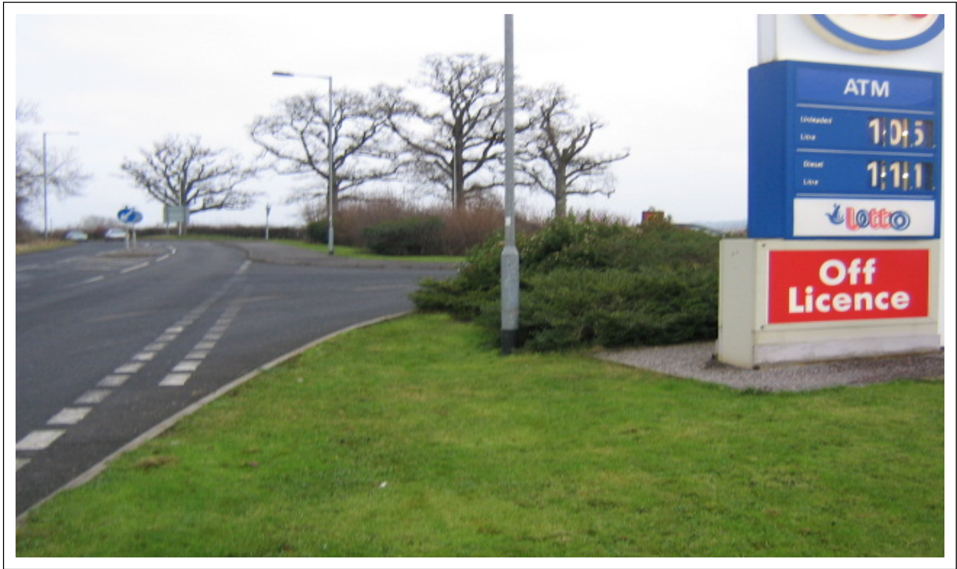
P0001 – No suspect materials observed to newer lamp posts at filling station access road
