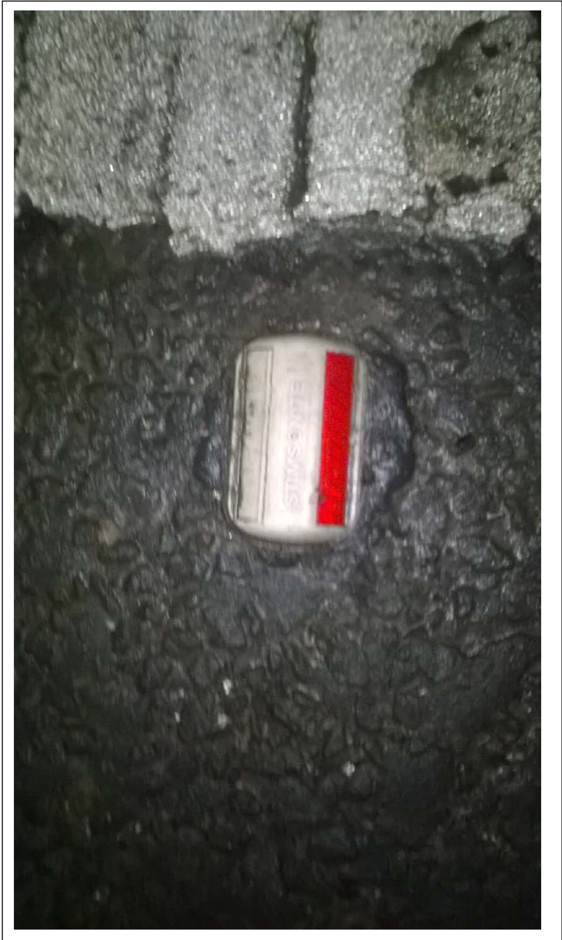
P0004 – Bitumen to deck W/B
